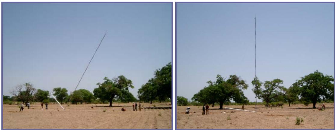
The 20m pole raised at an angle of 45°, with an electric winch (left) ; The pole is raised to vertical (right).
