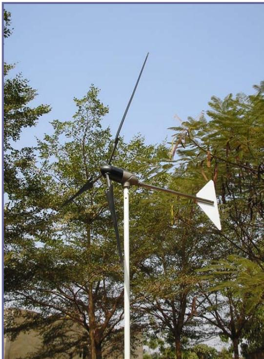
Before the installation in Karangana, the equipment was assembled for testing at MFC's office in Bamako. The installation was completed in May 2005. The wind turbine is rated at 1kW, and will be mounted on a pole of 20m height. The wind turbine is combined with an array of 1kW solar PV system. The two sources of energy are complementary to one another depending on the availability of wind and solar radiation.
