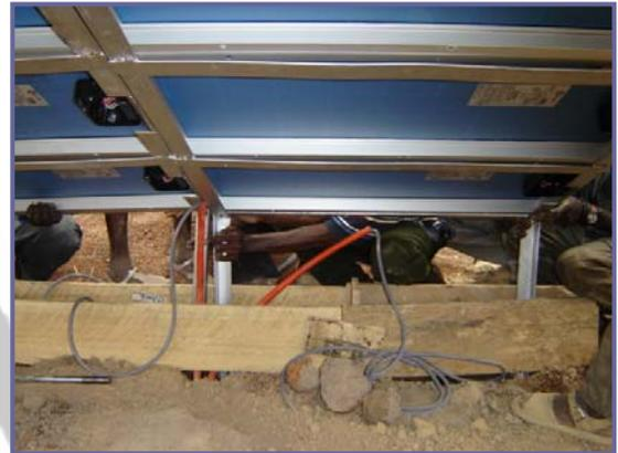
*Fig. 5. Putting the frames in the concrete foundations for a battery charging installation. Fig. 6. setting cable duct into the concrete to allow secure and longlasting electrical connections.*
