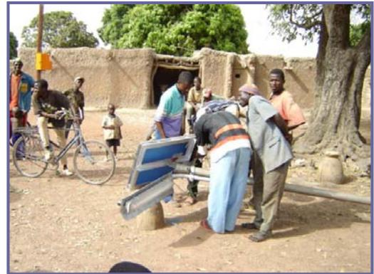
*Figs. 1 & 2. Making the electrical connection of a 50W panel for the solar lamp post. The lamp post can provide lighting from dusk until midnight for meetings, village celebrations and improved security.*
